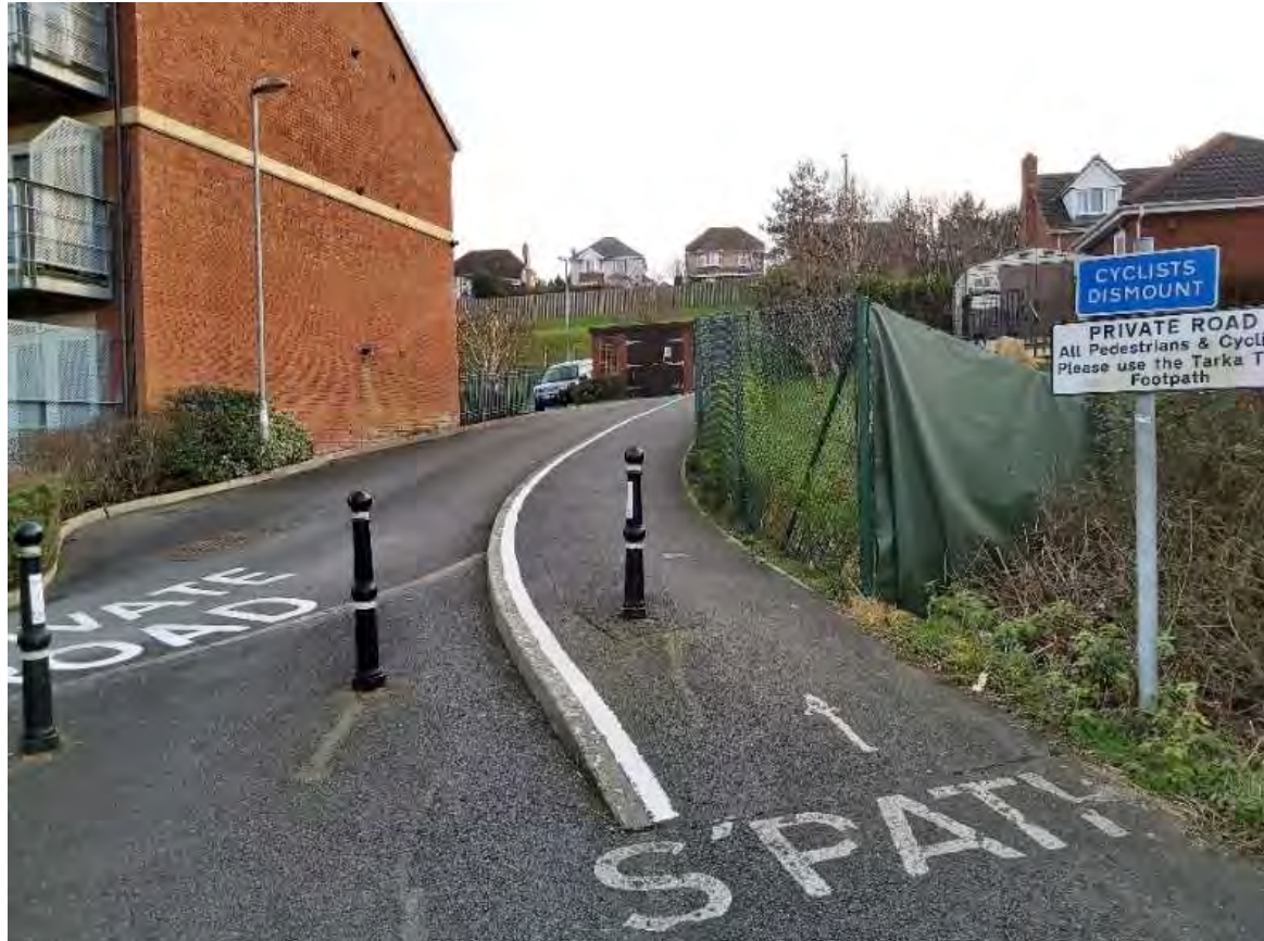
Figure 5-2 - Examples of barriers which could limit access to cycle users
